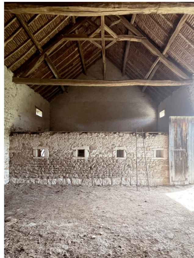
Former state - Central area
